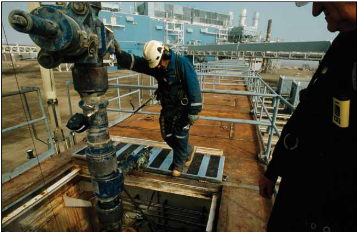
Oil workers perform a 'work over' on a thirty-year-old well head in Prudoe Bay.
