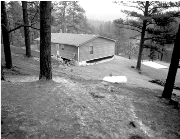
Figure 5. Following "firewise" principles, the owner of this home removed fuels within its "home ignitability zone" in the West Creek Subdivision, Colorado. As a result, it survived a crown fire in the wildland-urban interface during the 2002 Hayman Fire in the Pike National Forest. Photo © Karen Wattenmaker/kwphoto.com.
